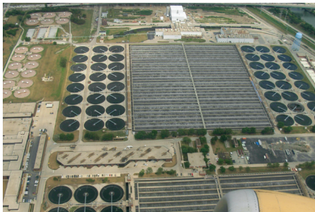
Stickney Water Reclamation Plant
